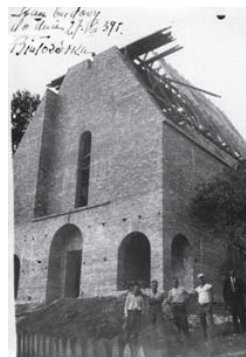
Fig. Construction of the church in Białozurka. As of August 27, 1939. ADŁ collections
